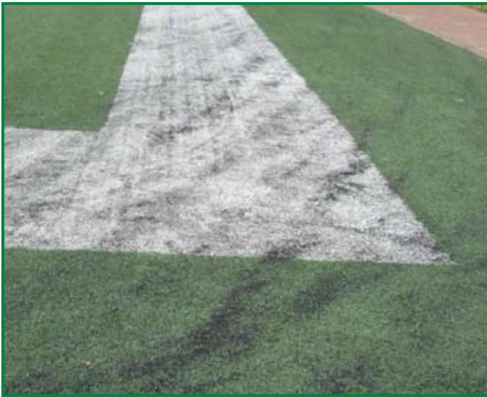
Figure 3: Ambient rubber infill migration towards the extremity of this all rubber field.
