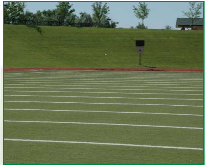
Figure 4: The FieldTurf at Dick Bivins Stadium is 10 years old! It consists of a Cryogenic rubber and silica sand layered infill. Even after 10 years there exists no signs of infill migration!
